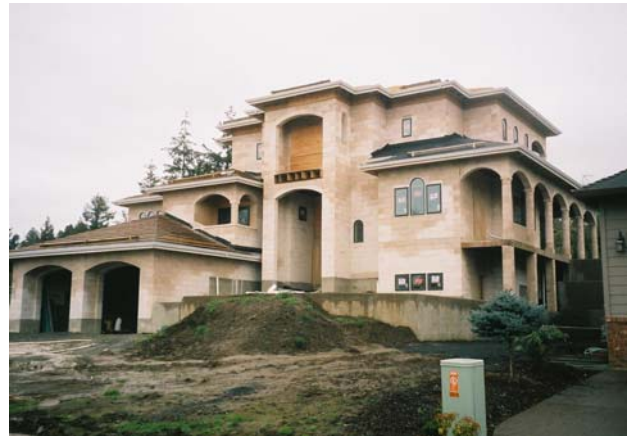
Home designed with E-Crete. Courtesy of Cascade Stone Craft
