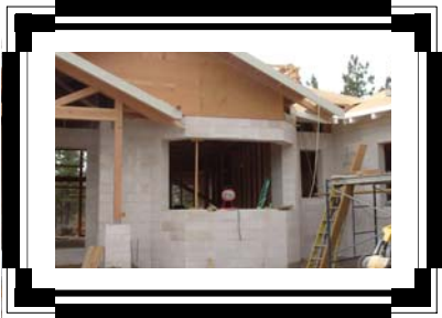
Hamond Residence—AAC Block
